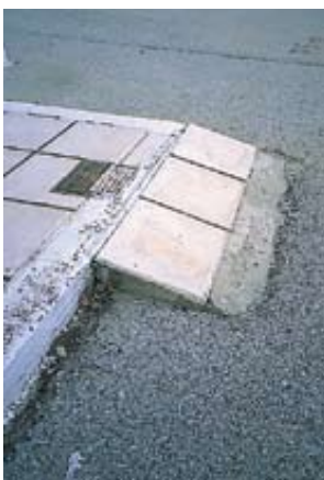
Unsuitable ramp, gradient steeper than 10%, the sides uneven (dangerous for pedestrians, Thessaloniki, 2005).
