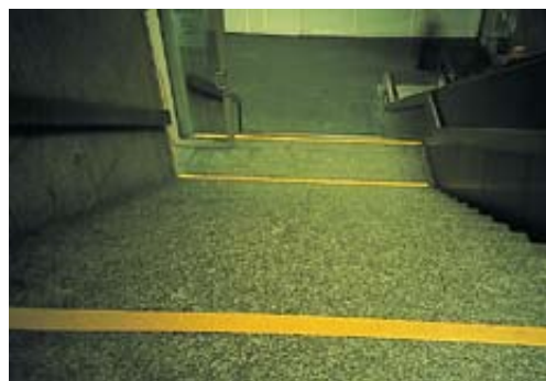
It can be hard to see where each step begins and ends, so yellow strips along the edge of each step are essential for safety (Steps leading to Brussels underground railway, 2003).
