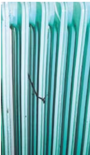
Radiator held in place with wire – a makeshift and dangerous arrangement (Thessaloniki, 2005).
