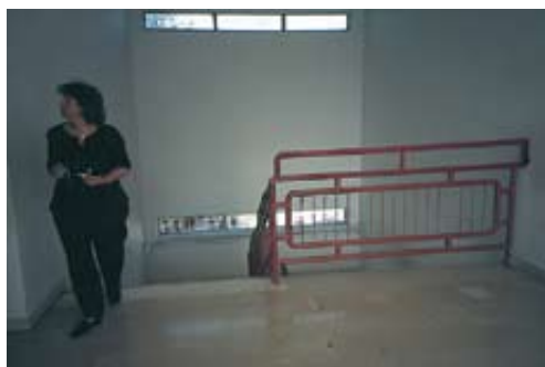
A common sight in Greek schools – the original rails were too low and have had to be raised.
