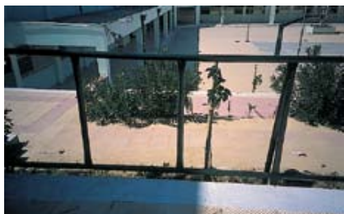
Insecure handrail and railings, with large gaps (Patra, 2002).
