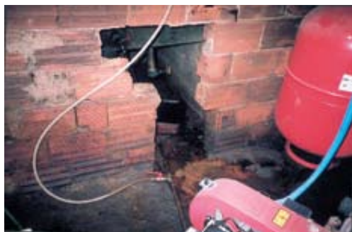
A dangerous state of affairs – leaking heating oil and a breach in the wall surrounding the fuel area (Thessaloniki, 2005).
