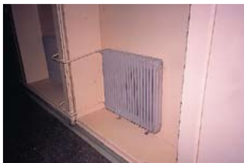
Installing radiators within a recess in the wall can prevent accidents (Thessaloniki, 2005).
