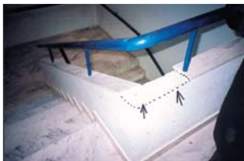
The marble (arrow) pieces should be fixed in place with special screws, not adhesive (Thessaloniki, 2005).
