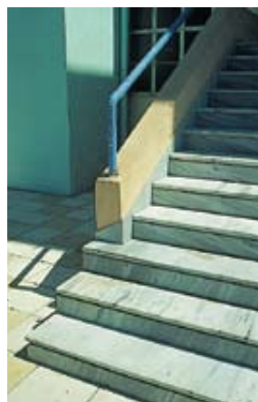
Here the handrail needs to be provided with something to prevent sliding, and should be extended right to the bottom of the stairs.
