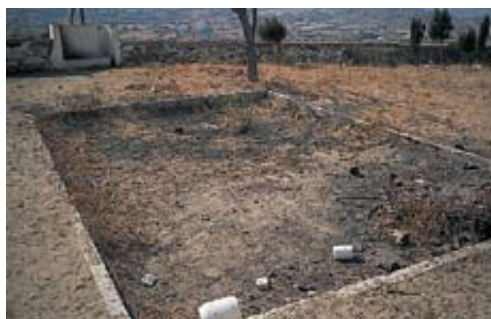
The sand in this pit is not being cleaned regularly. All too often in Greece the sand is neglected and allowed to solidify, causing danger of injury (Naxos Island, Greece 1991).
