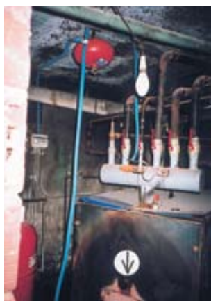
Note how the boiler (arrow) falls outside the range of the sprinkler. The arrangement inspires little confidence in respect of safety. The reader is reminded of two key points in the safety specifications:
