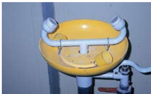
An eye shower (the student leans forward with his eyes between the two jets of water; the flow of water is operated with a pedal) for use when the eyes have come into contact with chemicals. This photograph was not taken in a school lab.
