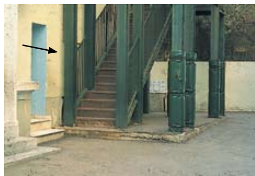
A job left unfinished! Note how only some of the columns have been sheathed in protective padding – an essential safety feature around stairways (Athens primary school, 2005)
