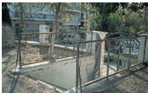
Note how the sides of the stairway are properly protected (Nafpaktos, 1992).
