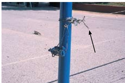
In all our travels we have hardly ever found a volleyball net properly suspended. Note the danger here from projecting ends of wire (Patra, 2001).
