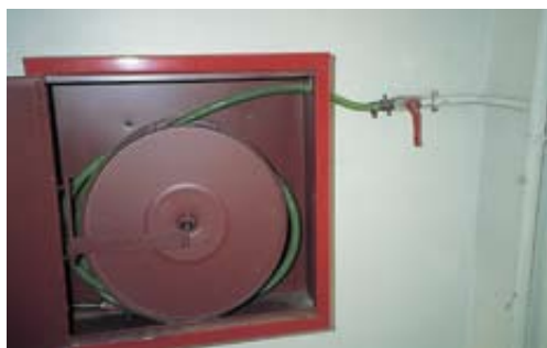
Note the narrow diameter of the hose – providing far too weak a jet of water in case of fire.
