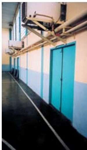
Note the dangerous position of the air conditioning units in this indoor gym (Thessaloniki, 2005).
