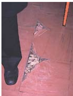
Dislodged floor tiles and tiles with curling edges are a common cause of falls (Thessaloniki, 2005).
