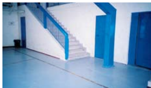
Poor design: note how the stairs and stair-rails are much too close to the playing area, and how there is no protective material around the basket support (Thessaloniki, 2005).
