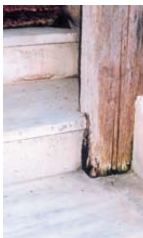
Note how this wooden post, supporting a roof, is beginning to rot (Thessaloniki, 2005)
