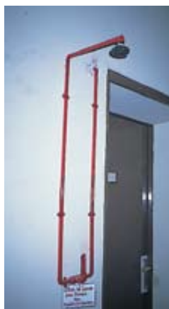
Full-size shower outside rooms where chemical substances are used (University of Athens, Medical School).
