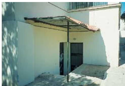
Note how the support for this overhanging roof is quite inadequate.
