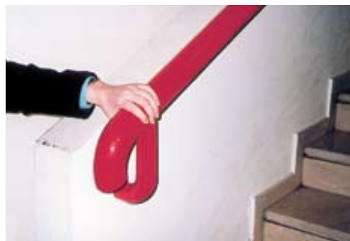
The diameter of the handrail is too large for a child's hand to grip. The ideal diameter is 3cm (Thessaloniki, 2005).
