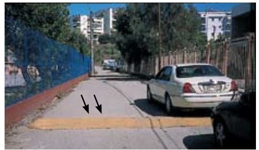
Road close to a school. Sleeping policemen should be designed to the proper specifications for height and curve; they should be clearly visible and there should be signs warning motorists of their presence! (A school in Patra, 2002).
