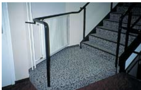
Note how the handrail goes all the way up the stairs from bottom to top. The stairs lead to a Brussels conference room.
