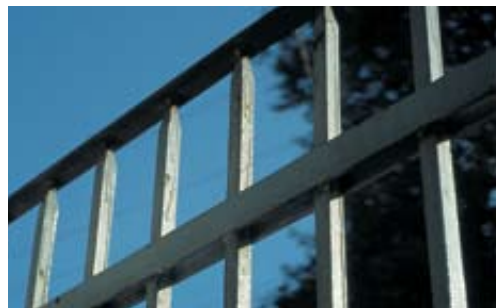
A good method of eliminating the danger of pointed railings (Nafaktos, 1992).
