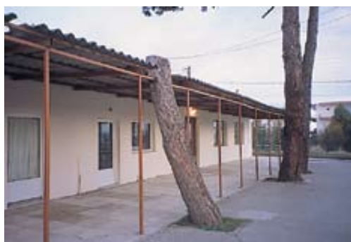
Dangerous roof made of asbestos sheets – cut with a saw to make room for the top of the tree! Asbestos should only be removed by qualified workmen (Thessaloniki, 2005).
