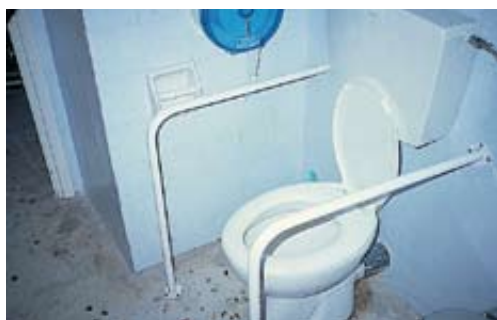
A WC with handrails for the disabled (University of Athens – Medical School).
