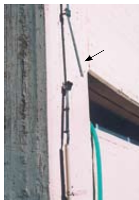
Damaged lightning conductor (Thessaloniki, 2005).
