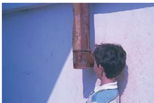
A rusting stove pipe ends just at the level of the children's heads, in the area where they play during their breaks (Philippiada, 1993).
