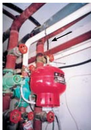
Here the fire extinguisher is suspended by a thin length of wire (Thessaloniki, 2005).
