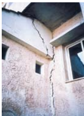
Dangerous crack in wall of school building, perhaps an example of earthquake damage (Thessaloniki, 2005).
