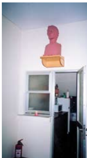
This bust could easily fall on someone's head during an earthquake (Thessaloniki, 2005).
