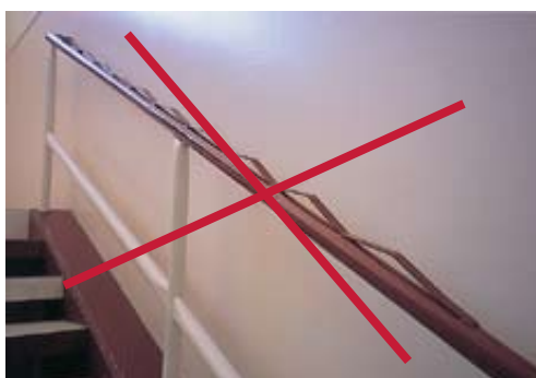
Definitely not the right way to prevent sliding – children's fingers might be caught under the strips of metal (Thessaloniki, 2005).
