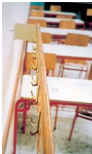
Fixing clothes' hooks on a length of wood facing the wall means they are less likely to cause injury (Thessaloniki, 2005).
