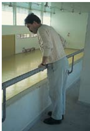
The balcony railing in this indoor school gym is dangerously low.
