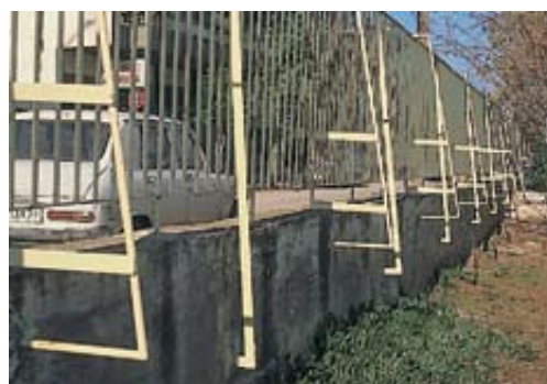
Dangerous projecting supports behind the railings of a school playground (Oropos, Attica, 1999).
