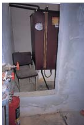
A wall about 40cm high surrounds the whole fuel area, even across the foot of the door (this is the correct arrangement - Thessaloniki, 2005).
