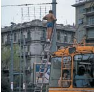
A scene showing a variety of violations of health and safety legislation: the ladder is set at the wrong angle and not properly supported, either at the top or the bottom; the workman is unsecured and is not wearing protective clothing, boots or helmet. And worst of all – the workman in the picture is setting up the loudspeakers for a rally organized by the General Confederation of Greek Labour!!!
